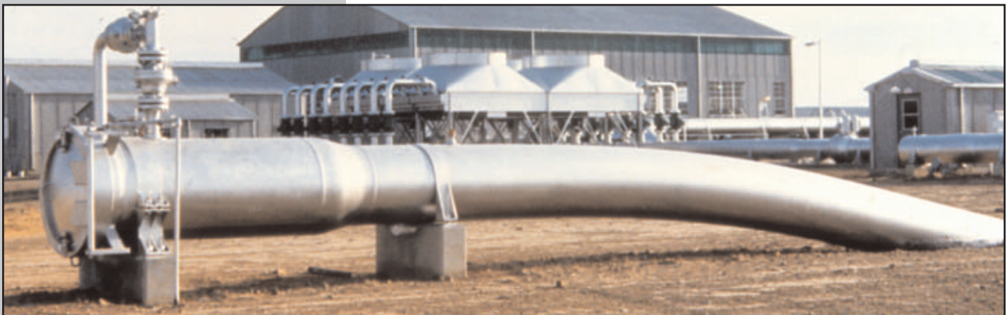
Typical of Tube Turns Yoke Type Hinged Closures being used with scraper traps.
